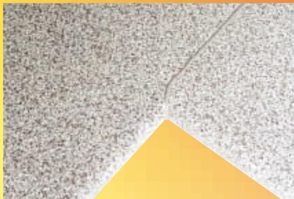
**Apply a liberal amount of Kolor-Bond to both sides of the joint to be sealed and bring surfaces together**
